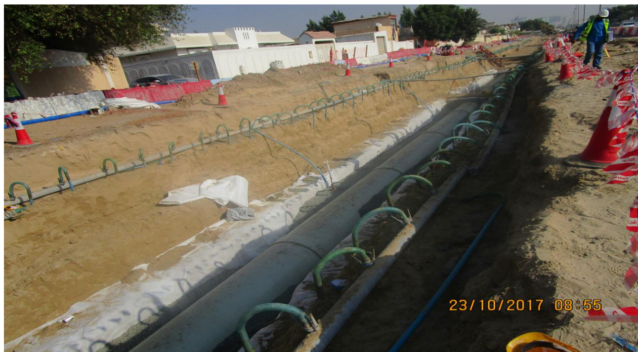
Laying of 1400mm dia GRP pipe
