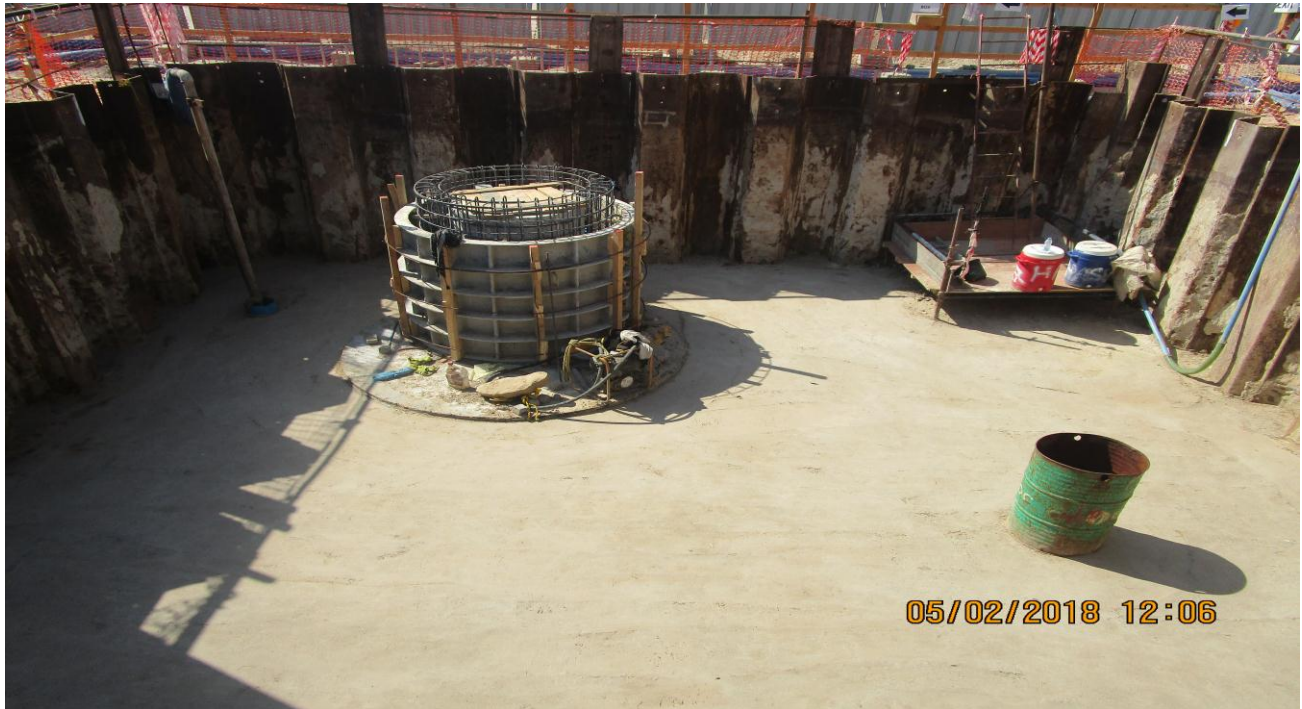
Construction of washout chamber at NDRC location
