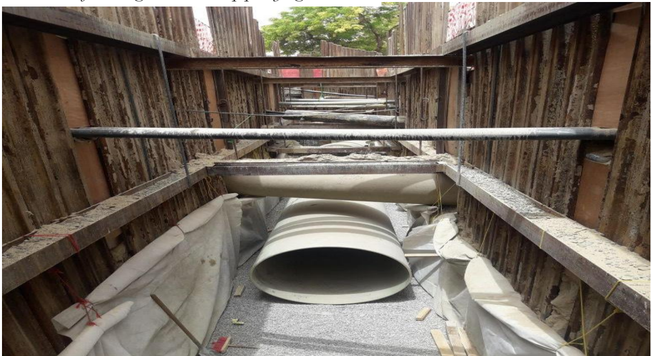
Protection of existing services while pipe laying
