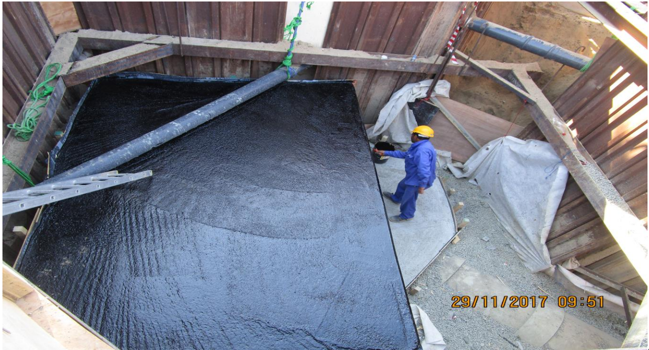
Application of tanking & water proofing
