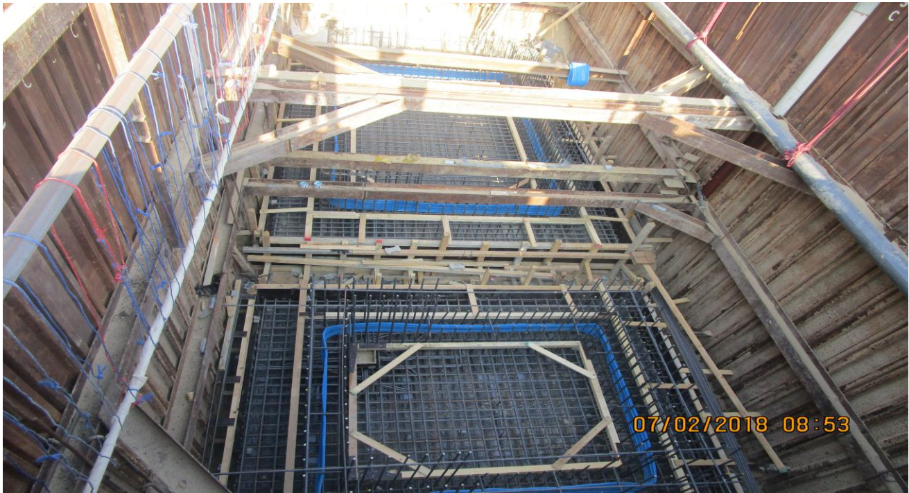
Construction of Flow meter & Isolation chamber
