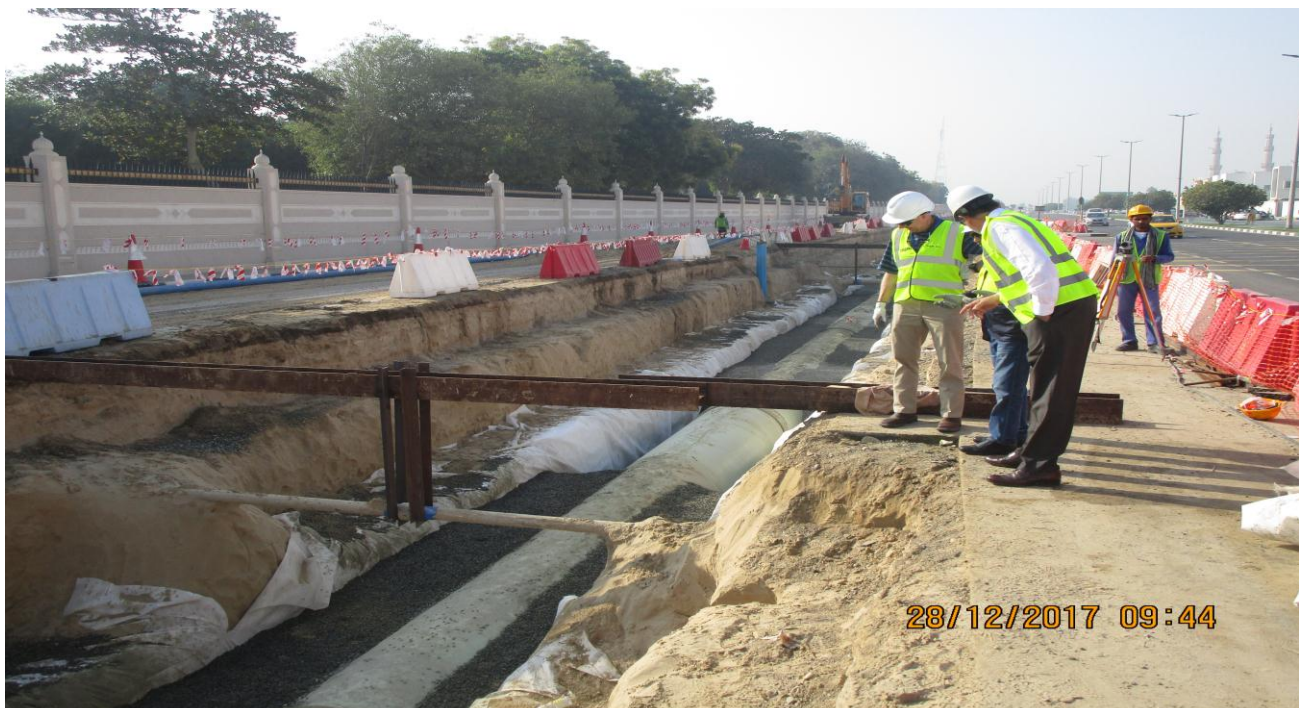
Laying of 1400mm dia GRP pipe
