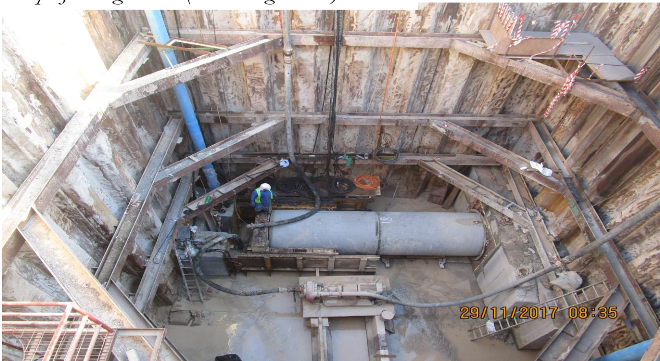
Pipe Jacking Work (Tunneling Work)
