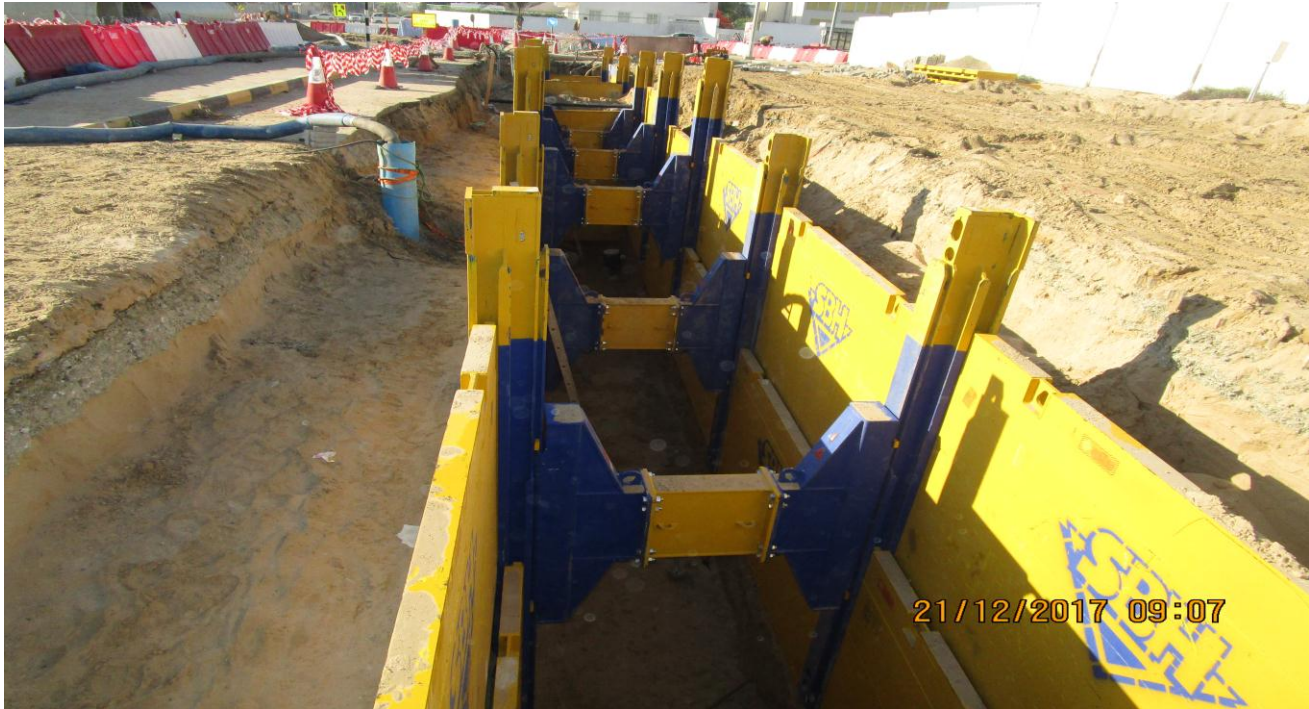
Fixing frame sheet for 1400mm dia GRP pipe
